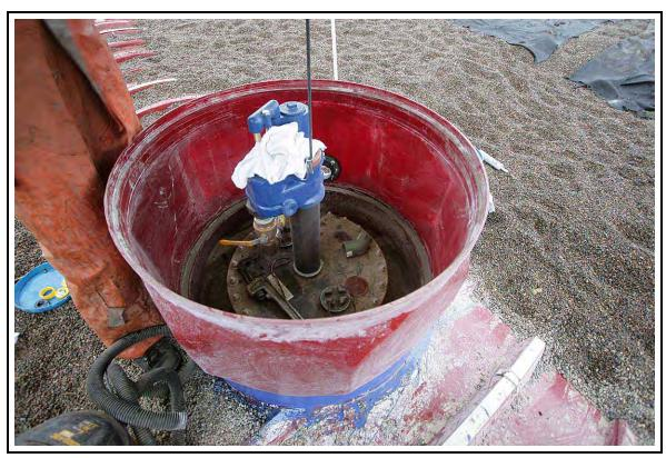
View of one of the three submersible turbine pumps and containment sumps being installed atop the underground storage tanks.
