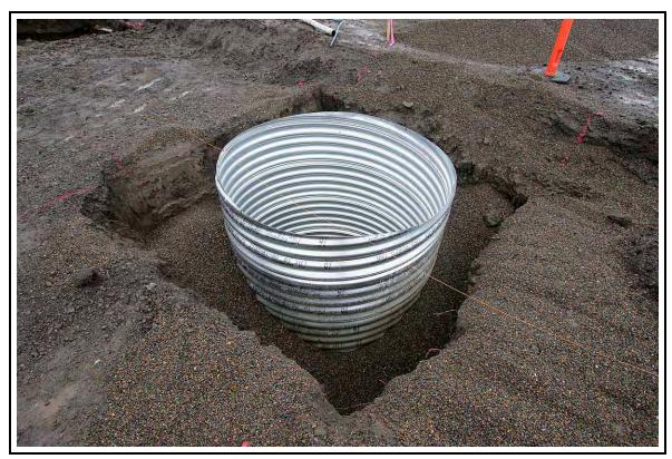
View of one of the six canopy footing forms being installed. Note that it is seven feet in diameter, which is substantially oversized relative to typical practices.
