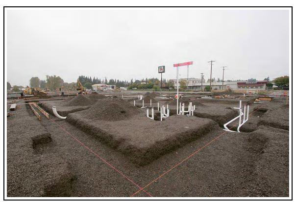
View looking southwest of the foundation excavation, foundation forming, and underground plumbing underway.
